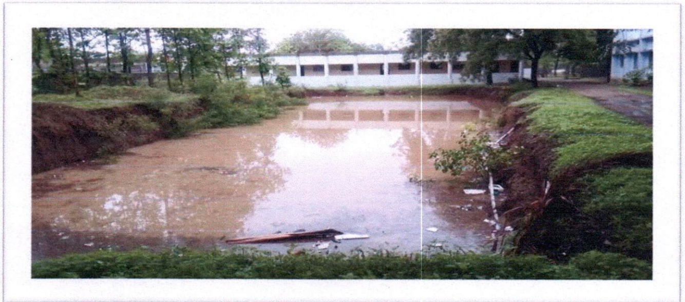
Check Dam Constructed in the campus
